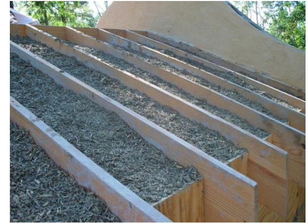
Hempcrete – roof insulation
