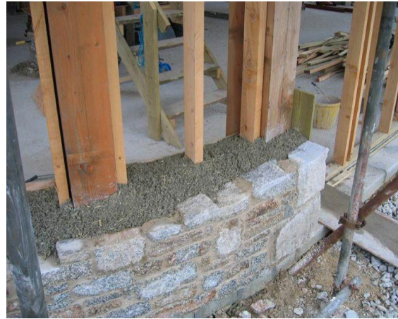
Hempcrete – cast around frame
